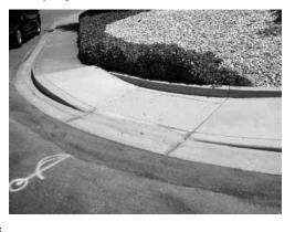
for pedestrians with physical disabilities along residential and commercial areas. They were built to be compliant with the new Americans with Disabilities Act (ADA) standards for accessibility. This standard requires new ramps to have a detectable warning surface mat on the ramp landing area that warns pedestrians with visual disabilities that they are about to enter a roadway with vehicular traffic. The project began in March 2007 and was substantially completed in July 2007.
